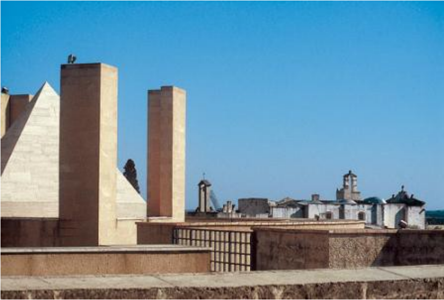
Fig.05 – Partial view of the chapel's roof
