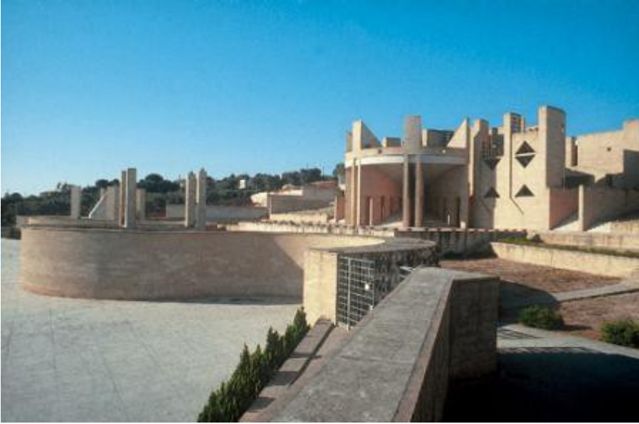
Fig.03 – View of the entrance and charnel house
