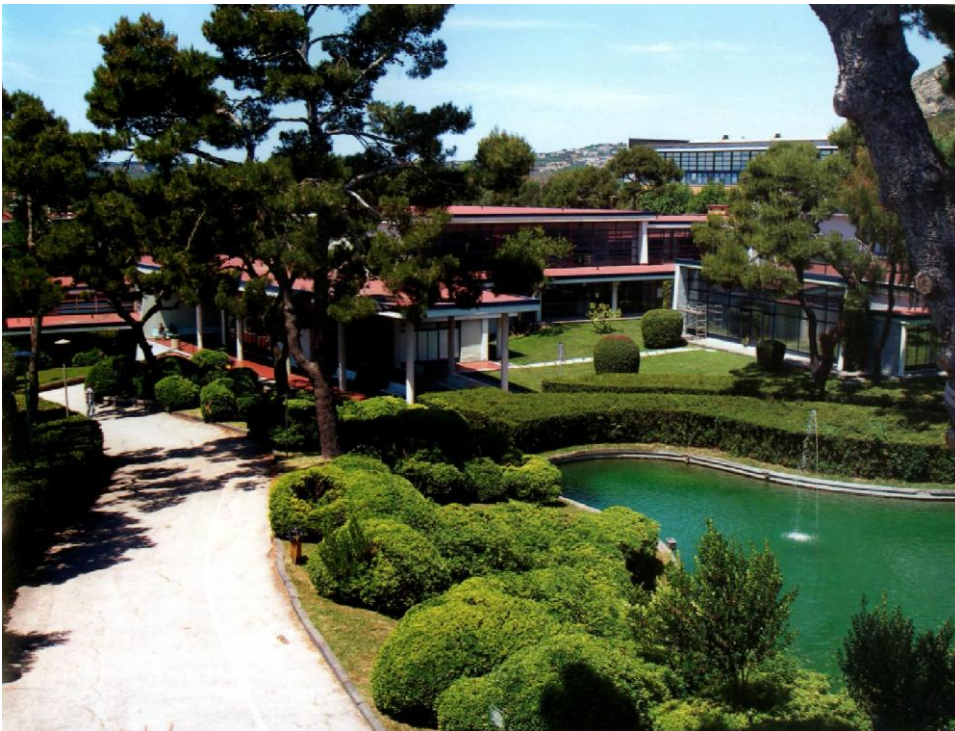
5.2.5 Social facilities nucleus, communal areas and tank (G. Cosenza (edited by), Luigi Cosenza. Fabbrica Olivetti a Pozzuoli , Naples 2006)
