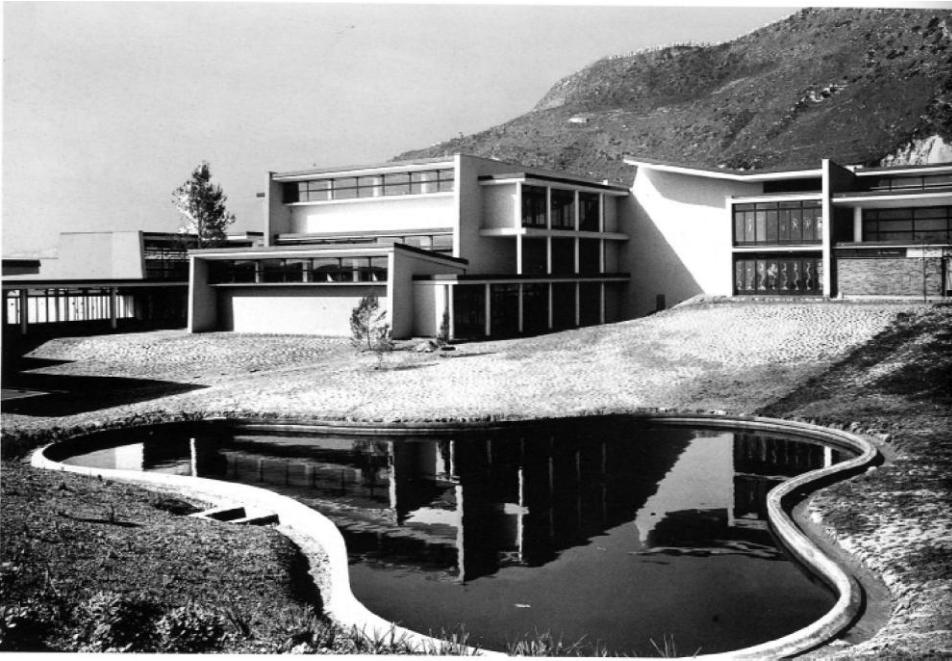
5.2.4. Tank, and link between workshop and changing rooms (G. Cosenza (edited by), Luigi Cosenza. La Fabbrica Olivetti a Pozzuoli , Naples 2006)
