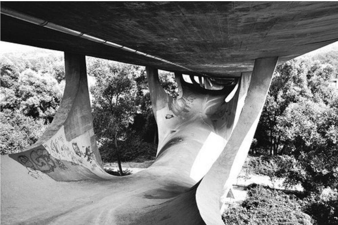
Fig.04 – View of the “covered walk”
