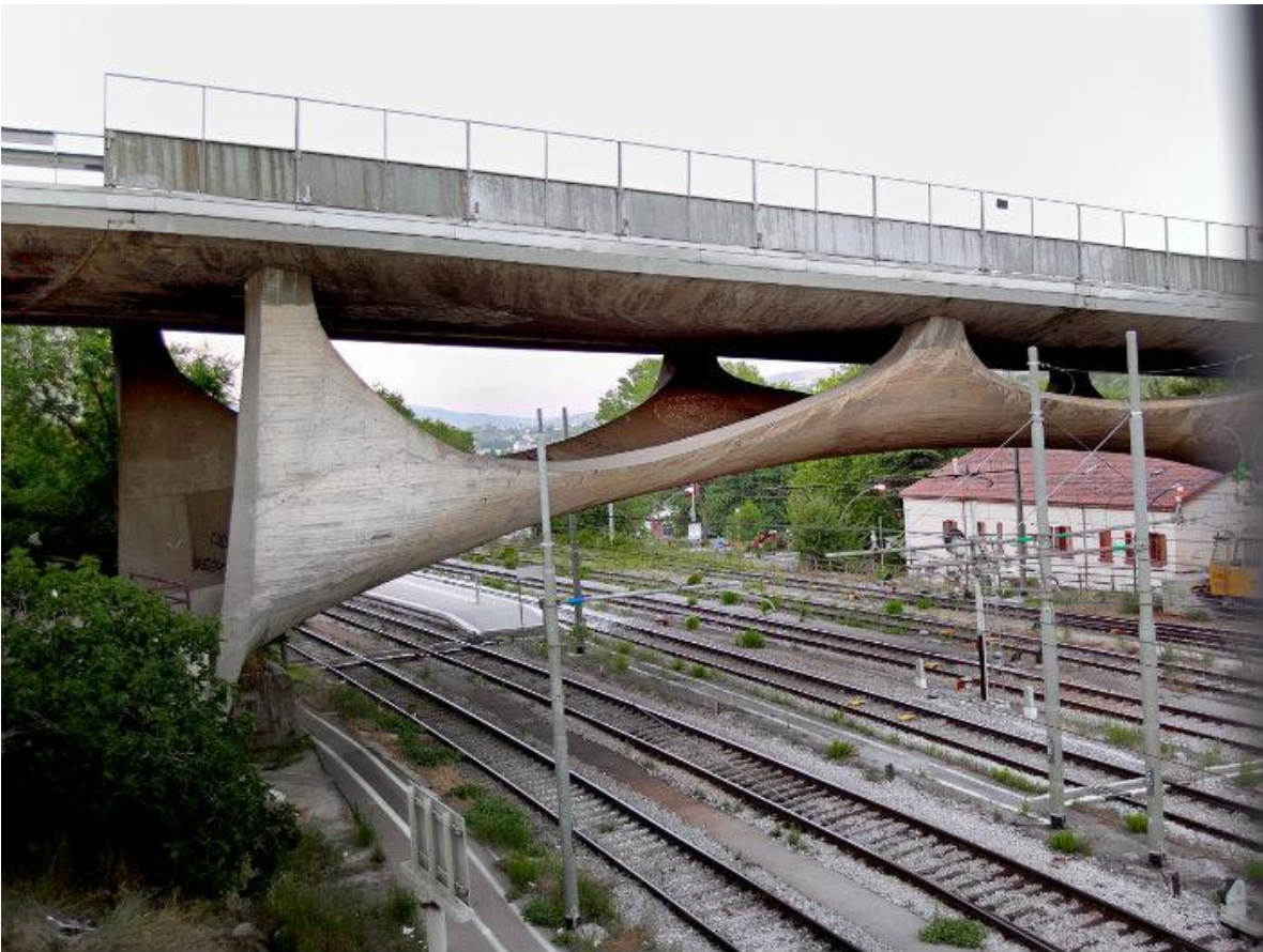
Fig. 02 – General view of the Basento Viaduct
