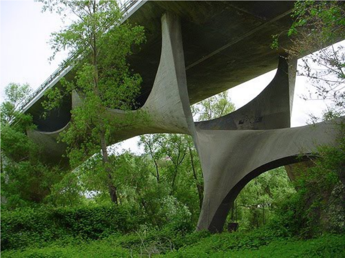
Fig.01 – General view of the Basento Viaduct
