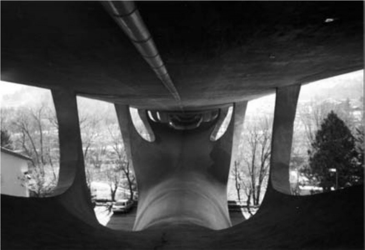
Fig.03 – View of the “covered walk”
