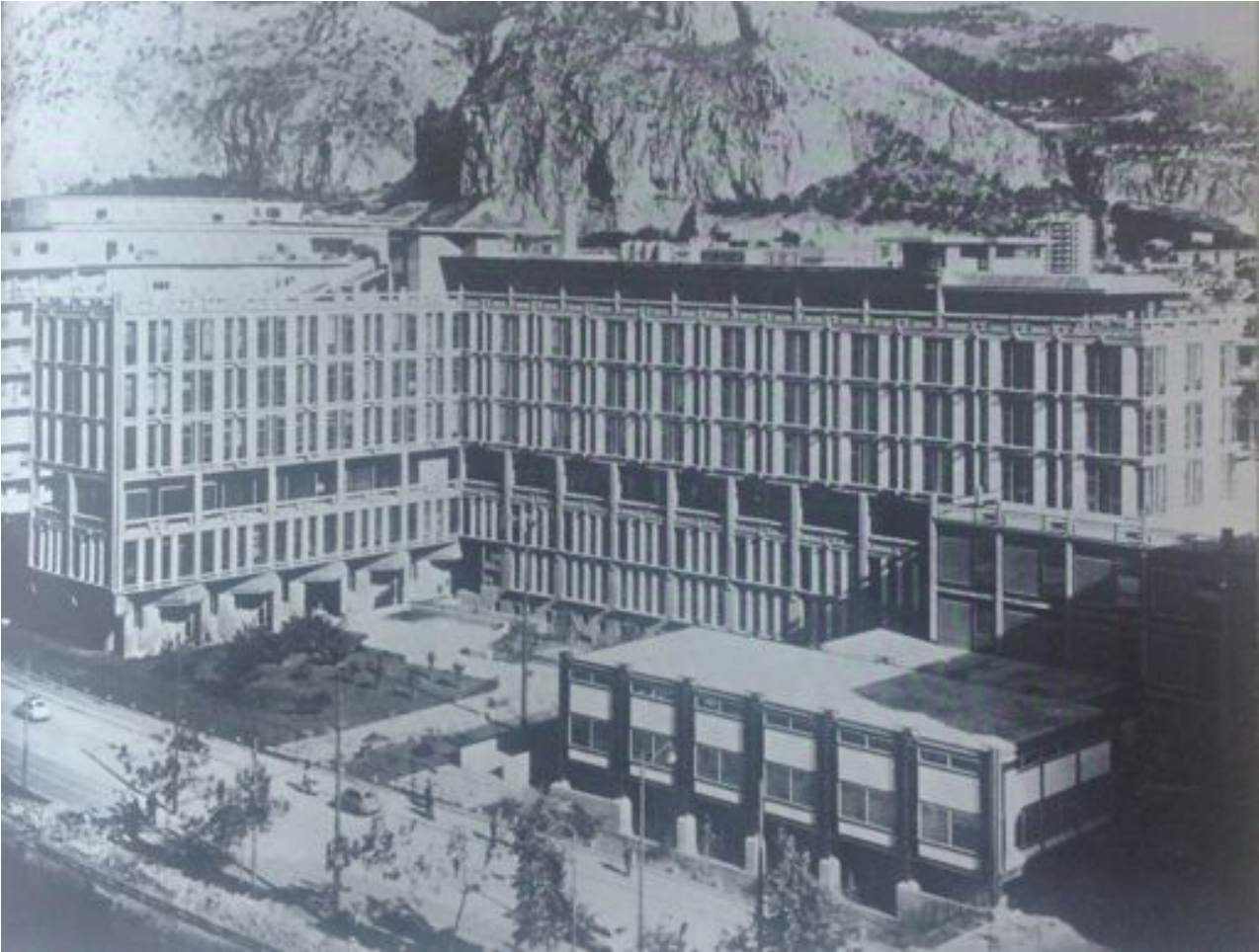
Fig. 3 General view of the building, about 1964
