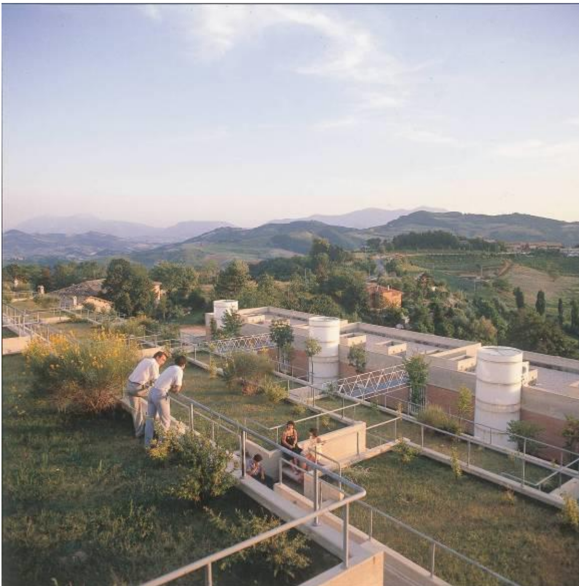
Fig. 13 La Vela, the terraces above the residential cells
