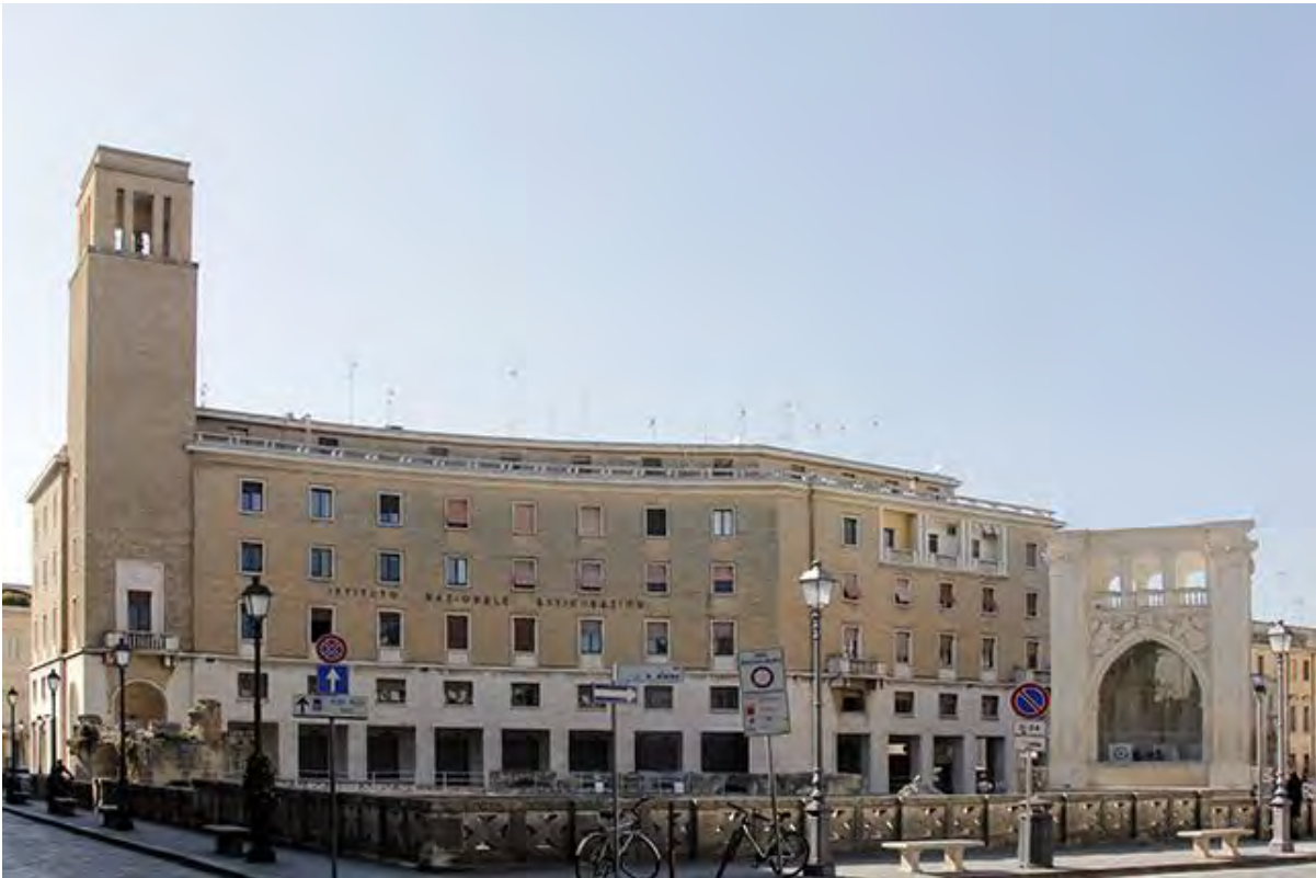
Fig.07 – Main facade on piazza S. Oronzo, 2020 (photo by Andrea Mantovano)
