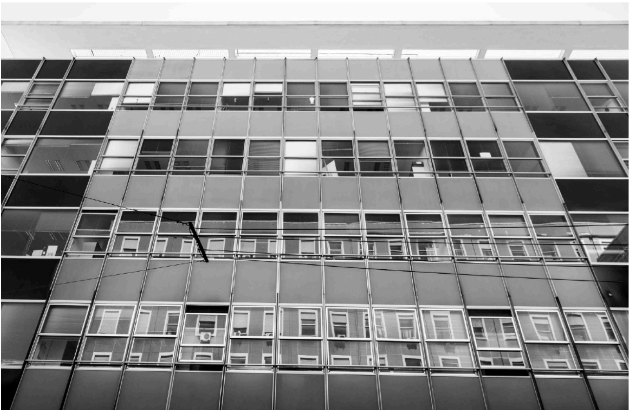
Fig.02 – Picture of the curtain wall (Adriana Maranghino 2019)
