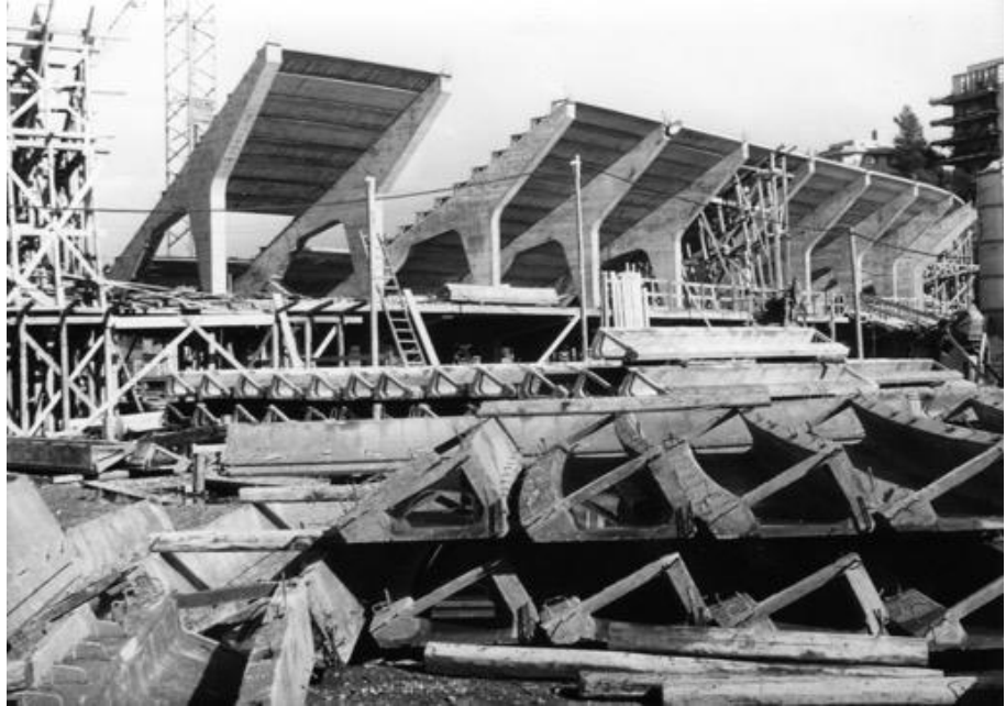
Flaminio Stadium construction site: precast seating units.
