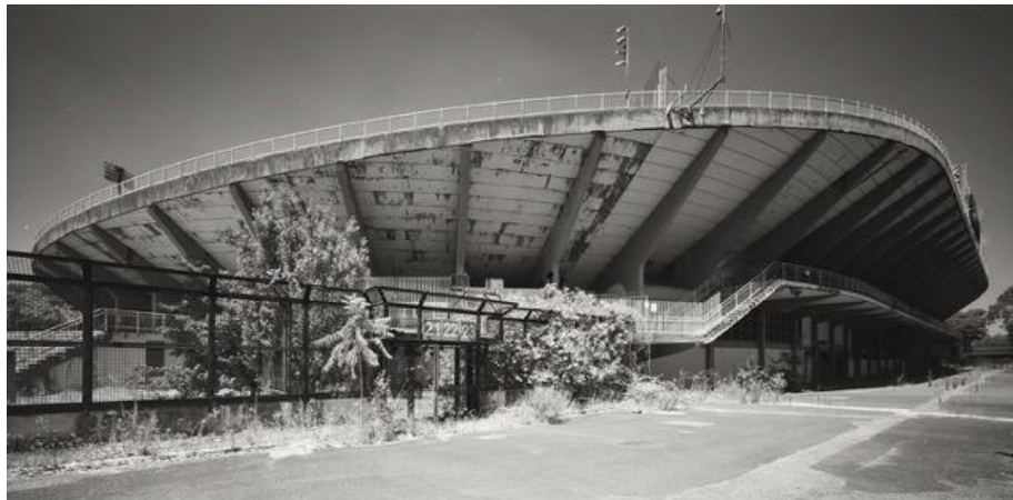
The Flaminio Stadium current state.
