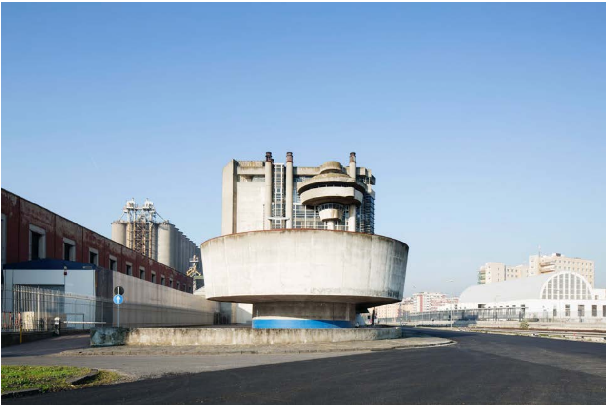
09_ The secondary façade for the south-East view in a dialogue with the Mercato Ittico designed by Luigi Cosenza on the right-side, 2017
