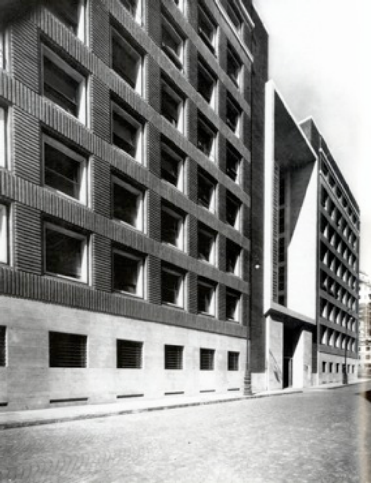
Fig 4 the front of the building
