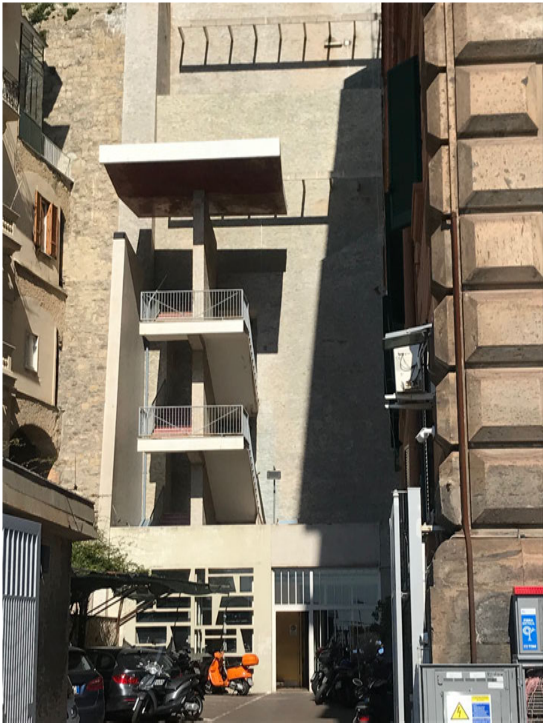
09_View of the the staircase in reinforced concrete, 2021
